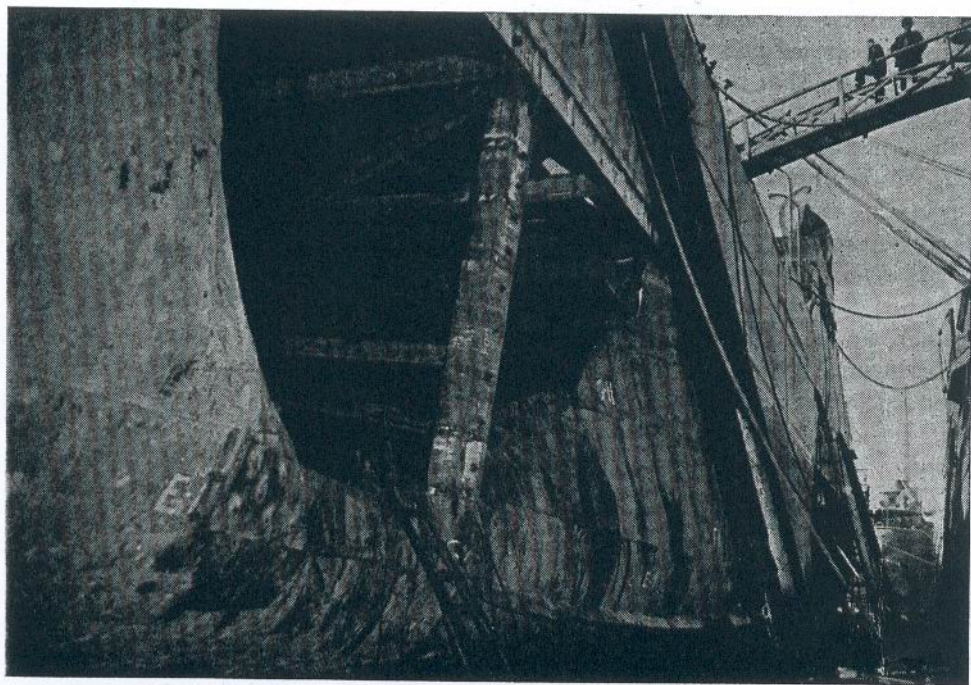
SAN ELISEO in dry dock at Barbados, May 1942.
